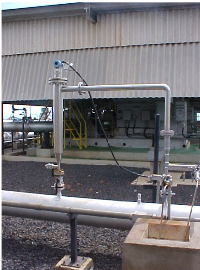
Figure 2.25 – Density measurement to identify the product
