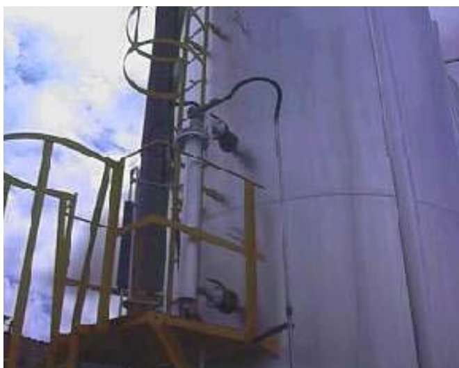
Figure 2.23 – Salt water/oil Interface Level Measuring
