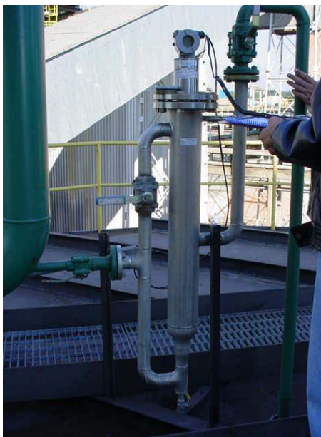
Figure 2.40 – Caustic Soda Concentration Measurement Installation
