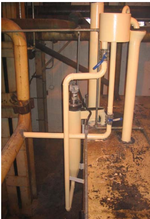
Figure 2.6 – Installation for Molasses Brix Measurement
