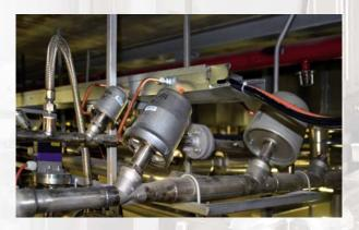
Alternatively to a convential solution with individual valves we can also provide manifolds, which save space, simplify maintenance and reduce heat losses.
